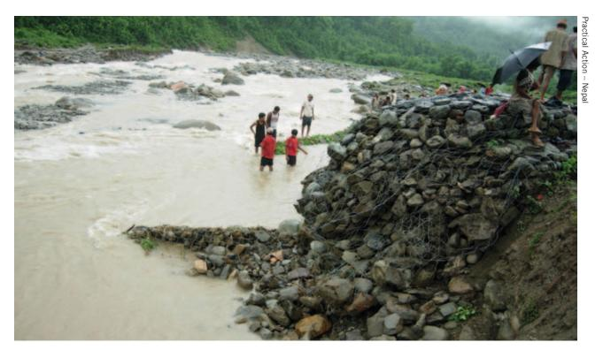
Repairing flood-damaged irrigation inlet
