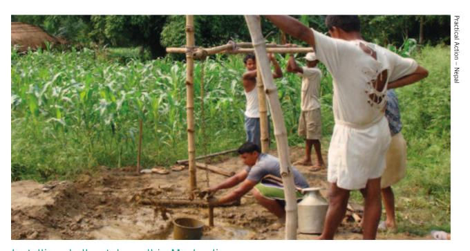
Installing shallow tube well in Meghauli
